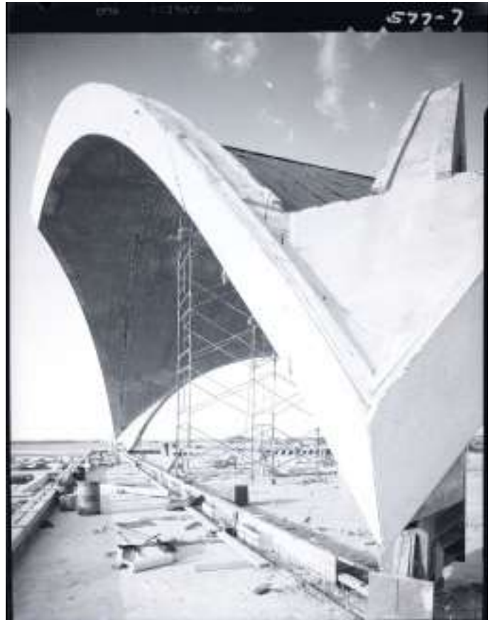
Concrete arches of the Lambert Airport terminal building under construction. July 15, 1954.
