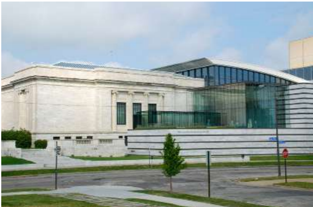
East facade, Cleveland Museum of Art's original building and new additions. Credit: Gary D. Sampson
